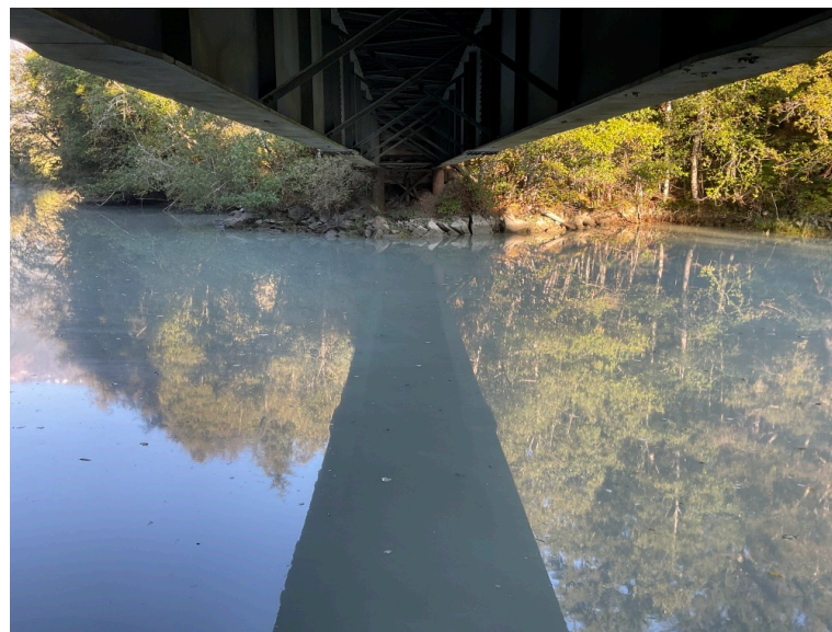
Left Bank Abutment when facing downstream
