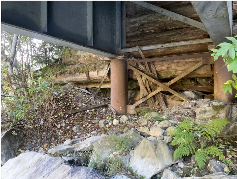
Right Bank Abutment when facing downstream
