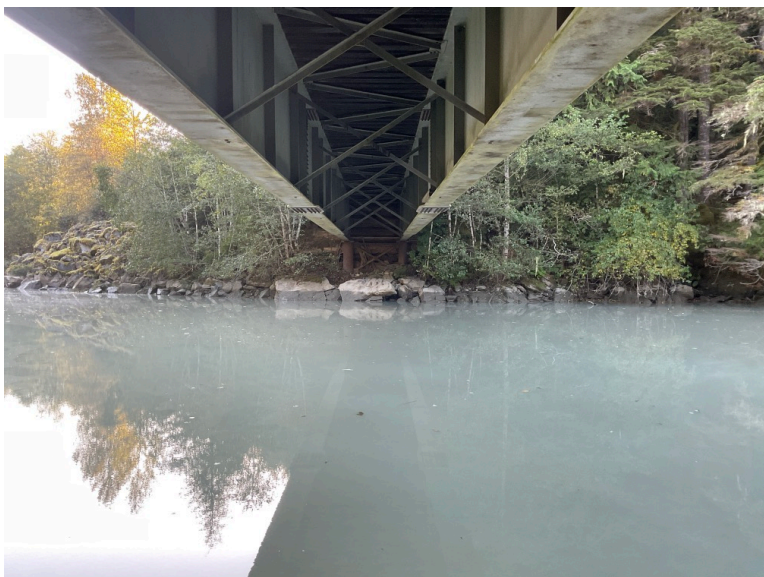
Right Bank Abutment when facing downstream
