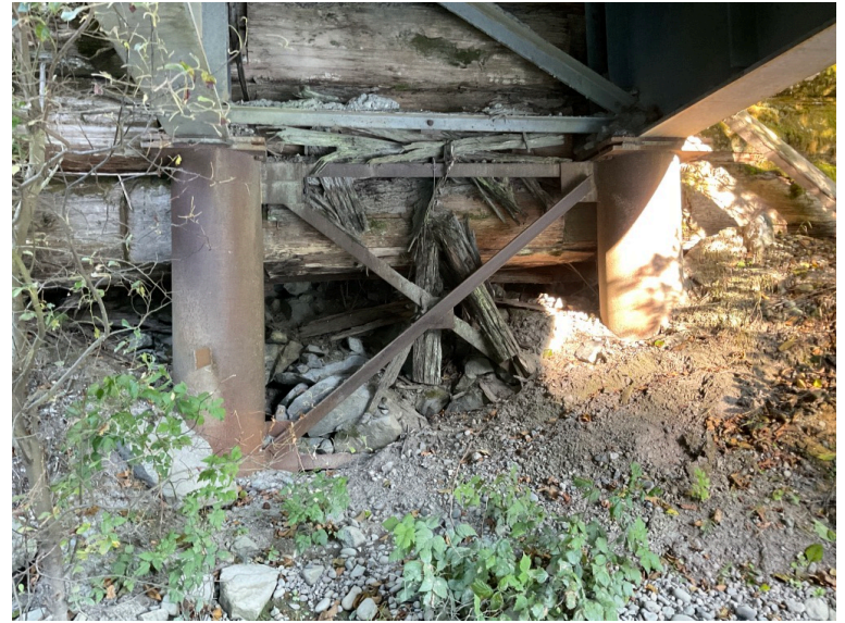
Left Bank Abutment when facing downstream
